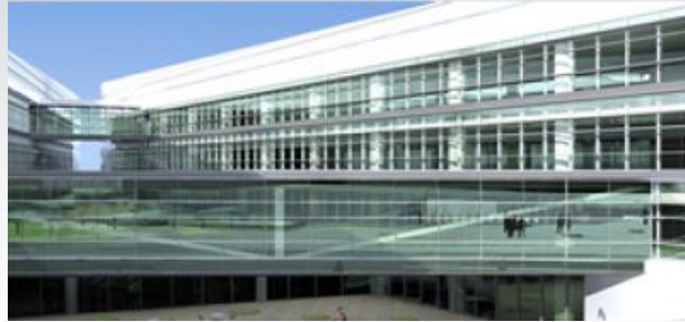
Sancaktepe Engineering Center (2015)
