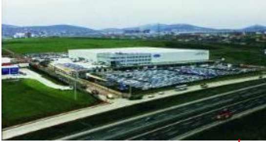
Sancaktepe Parts Distribution Center (1998)
