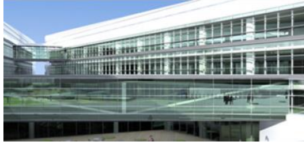
Sancaktepe Engineering Center (2015)
