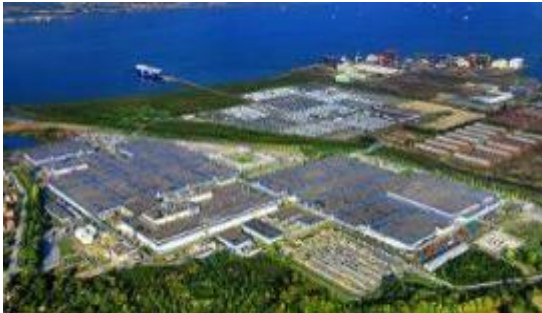
Kocaeli Plants: Gölcük Plant: Transit (2001), Custom (2012)
